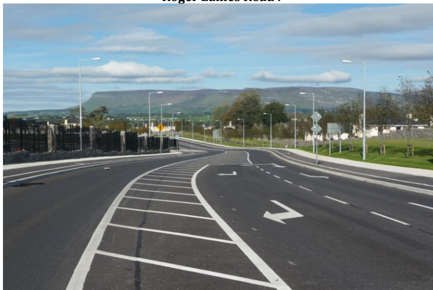
Western Distributor Road Phase 1 looking North towards the Strandhill Road recently named 'Roger Eames Road'.
